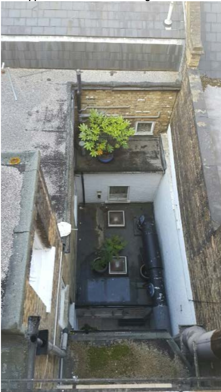
Photograph 2: View from upper floors of No. 19 Nottingham Place to rear of 4 Bingham Place
