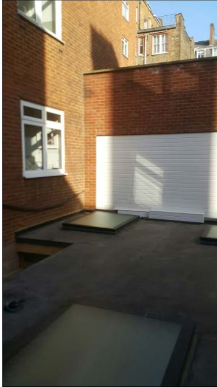
South (rear) elevation with newly erected lower ground floor extension in foreground
